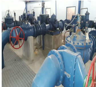
2 Water Pump Stations Repaired
