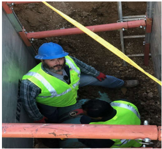
13 Water Main Repairs
